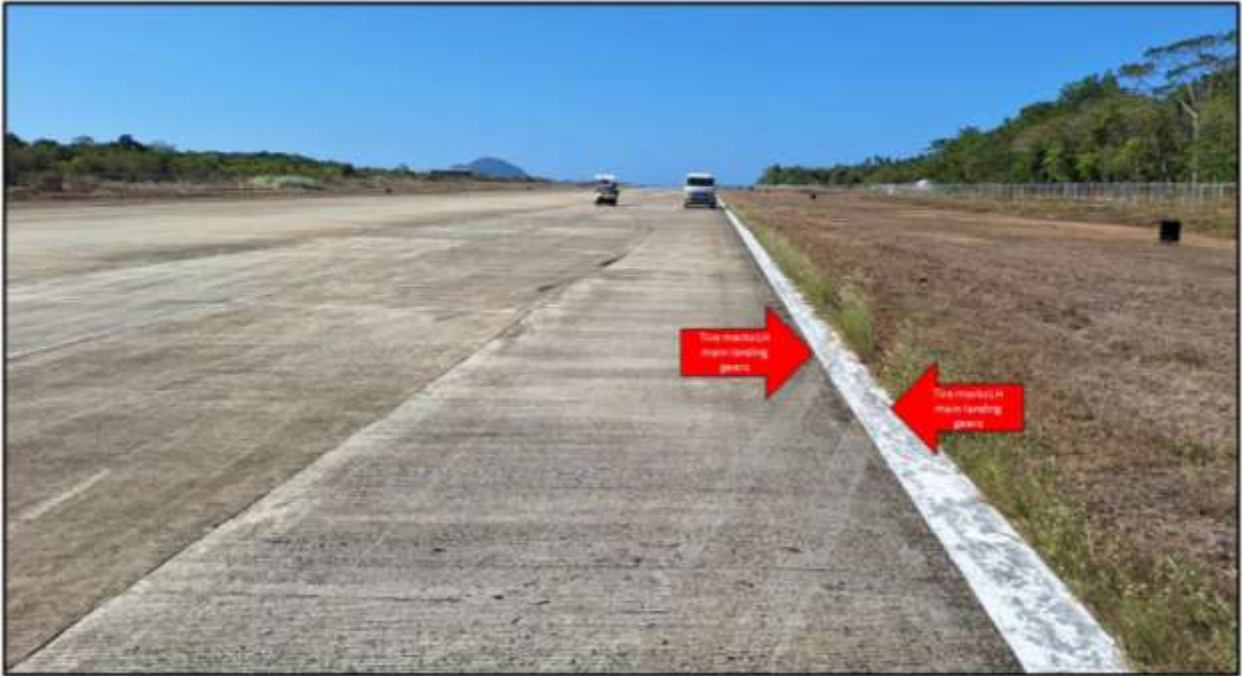
Figure 6 – Tire marks of the aircraft re-entering the paved portion of the runway.
