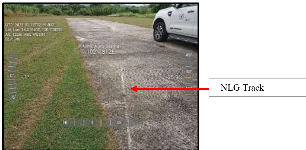
Figure 4: NLG scrape marks on the runway
