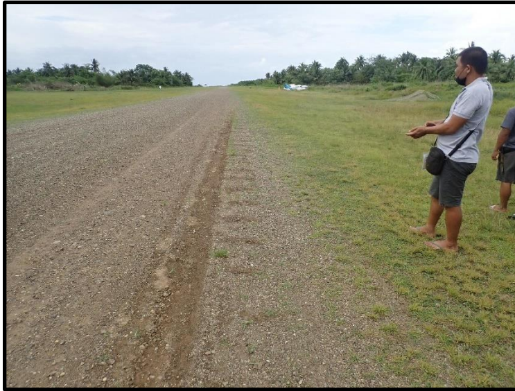
Figure 2. Multiple right-hand propeller scrapes on the runway.
