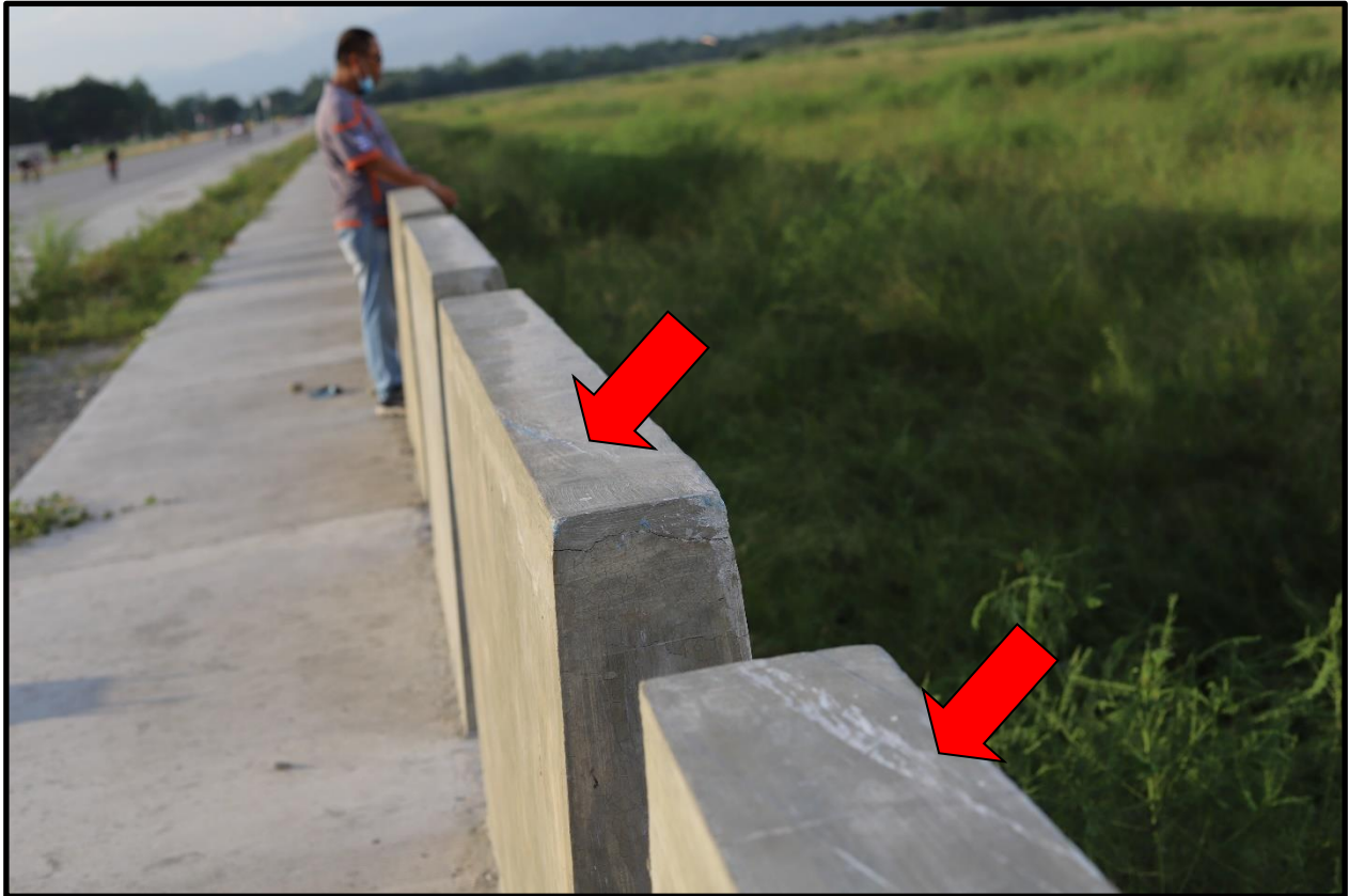
Figure 2 – Scratches on the roadside concrete barrier due to contact with the wing tip
