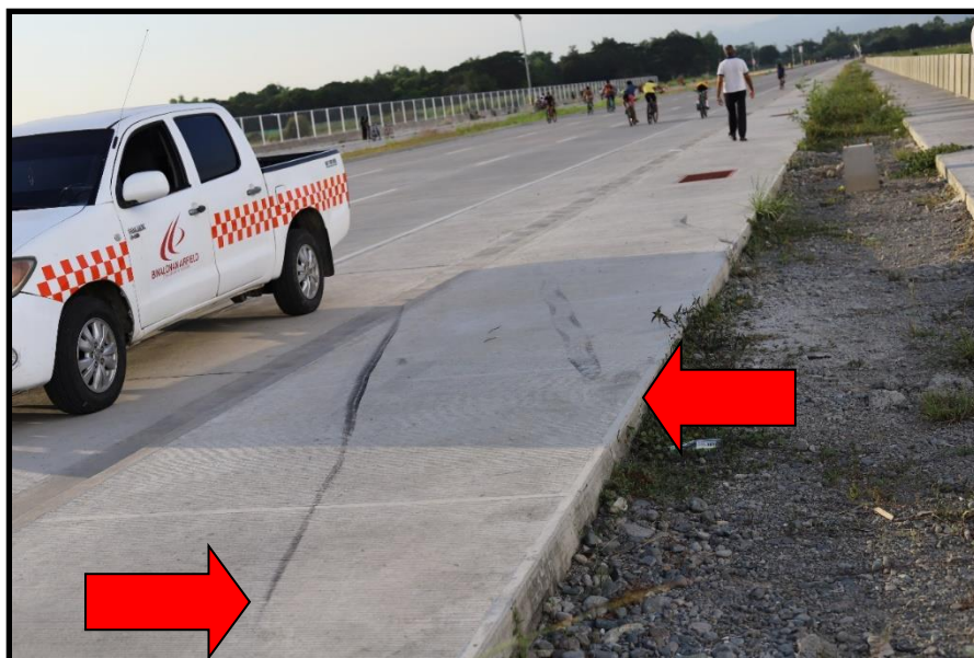
Figure 1 – Tire marks on the touchdown area of RP-C1028
