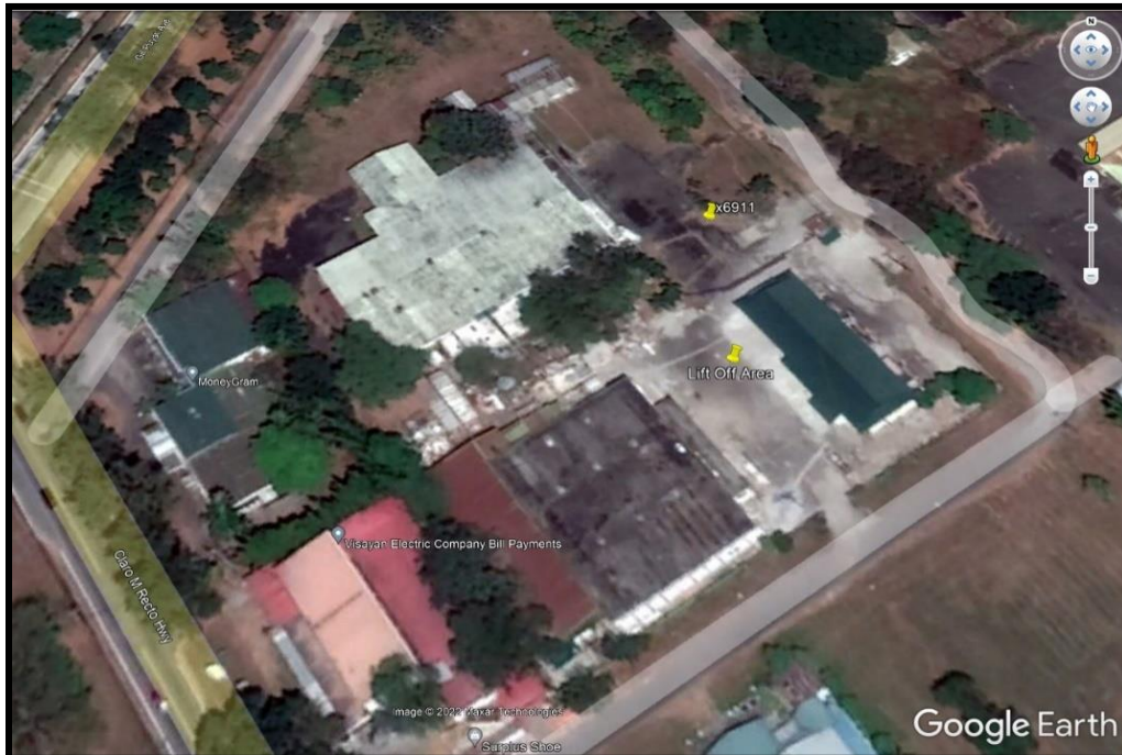
Figure 10. The helicopter lift-off and its final resting place is about 35 meters.
