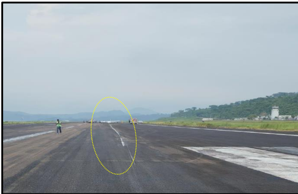
Figure 2 – The aircraft's touched down point and visible skid marks over RWY 07.
